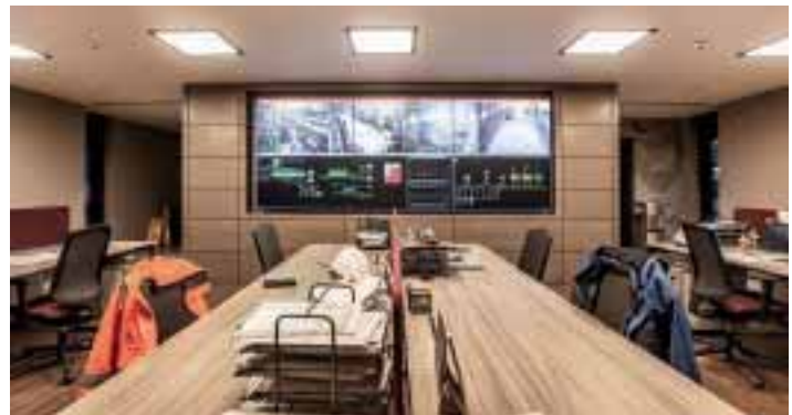
Displays in a 3 x 2 configuration can be found in the smaller control rooms, monitoring specific aspects of the facility's operations
